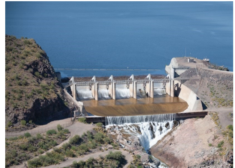
Horseshoe Dam Reservoir and Spillway
