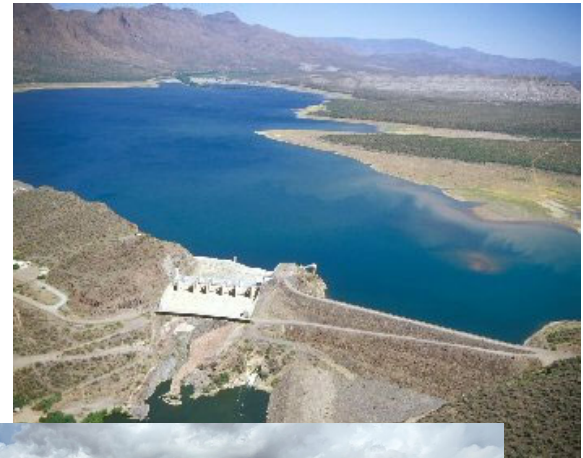
Horseshoe Dam and Reservoir
