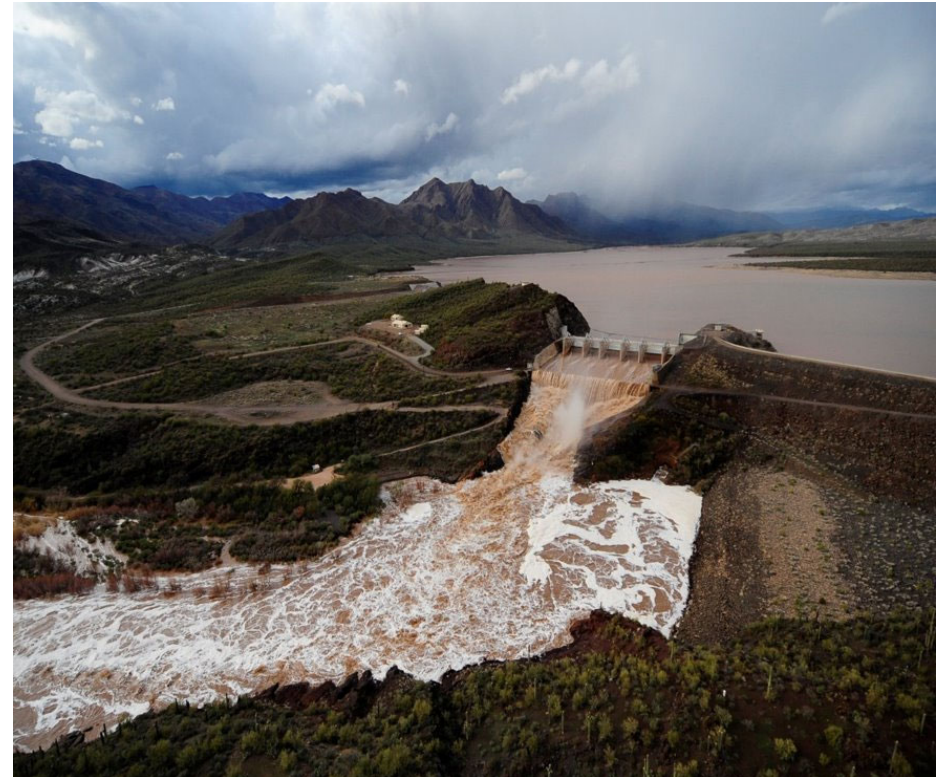
Horseshoe Dam Reservoir and Spillway
